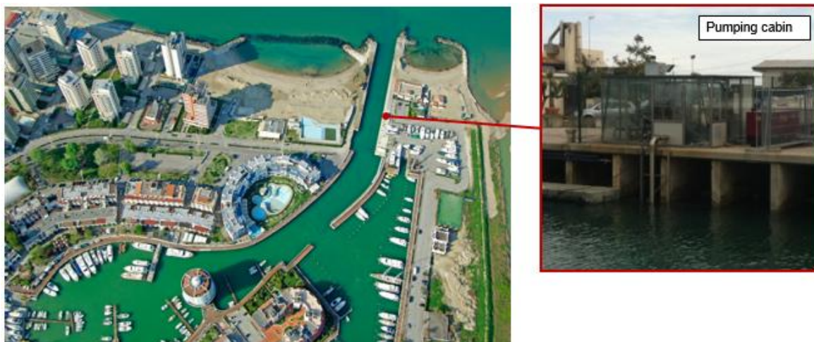
Figure 4: The installation in the harbor at Portoverde in 2012. In the left a schematic representation of the plant is proposed
